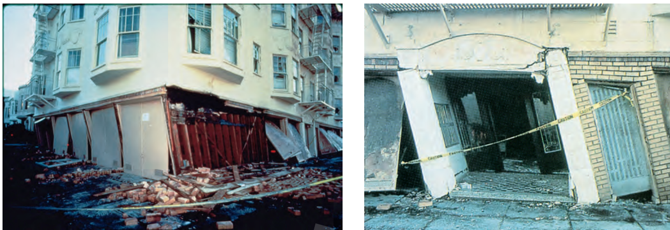
FIGURE 4.23 In general, structures anchored in bedrock have the best chance at surviving an earthquake, while those built on unconsolidated materials generally suffer the most damage. A case in point is the effect of the 1989 earthquake in Loma Prieta, California, on the city of San Francisco. In the downtown area, where the foundations of the buildings are in bedrock, there was little damage. Most of the damage occurred in the Marina District, where the structures were built on land formed by dumping the unconsolidated debris of the 1906 San Francisco earthquake along the edge of the bay. Photos: (left) Courtesy of J. K. Nakata/USGS; (right) Courtesy of C. E. Meyer/USGS.
