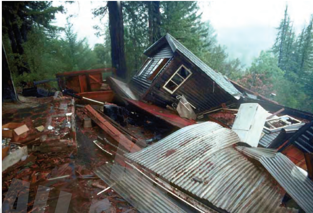
FIGURE 4.24 Love waves can literally move the foundation from beneath homes, as they did to this home during the 1989 Loma Prieta earthquake. Current building codes require that this type of structure be bolted to its foundation. Photo: USGS.
