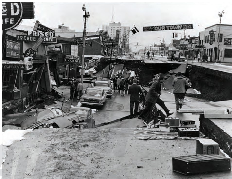
FIGURE 4.16 The largest recorded earthquake in North America occurred in 1964 in Alaska's Prince William Sound. The quake, which had an estimated moment magnitude of 9.2, destroyed downtown Anchorage. This photograph shows a graben that subsided 11 feet in response to 14 feet of horizontal movement. Photo: USGS; Map: Shutterstock 15180868, credit Map Resources.
